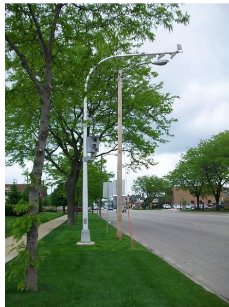
Figure 15. Red light camera equipment in Cedar Rapids, Iowa
