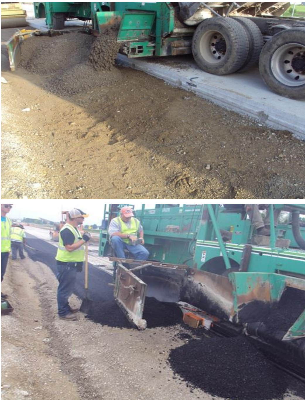
Figure 30. Shoulder construction: backfilling (top) and HMA shoulder paving (bottom)
