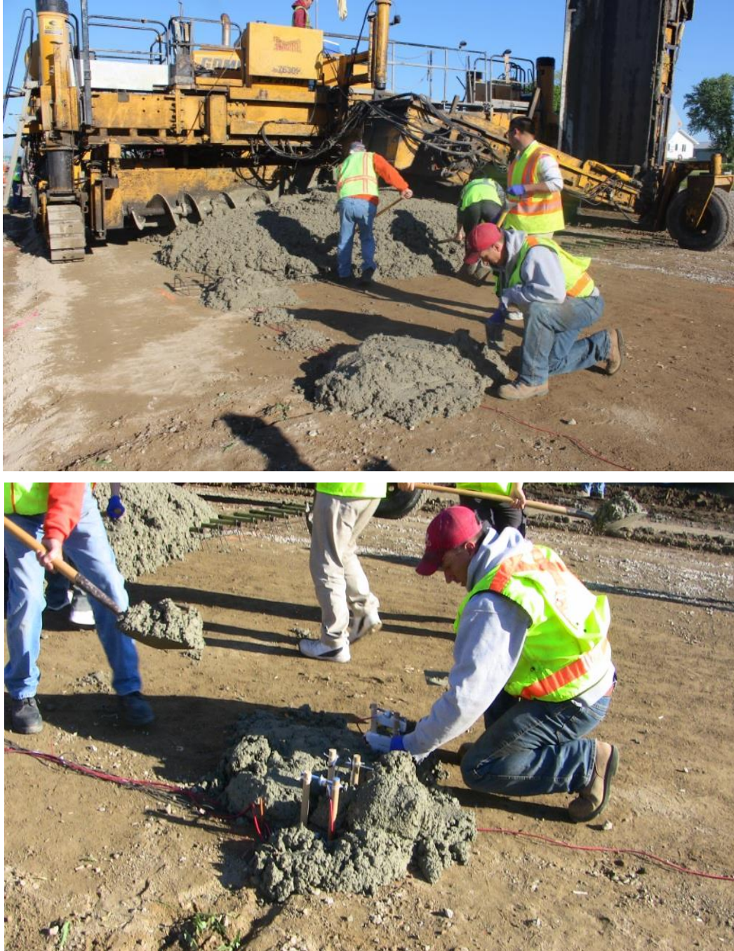
Figure 27. Sensor protection during road construction: obtaining fresh concrete from the paver (top) and pouring concrete on the sensors (bottom)
